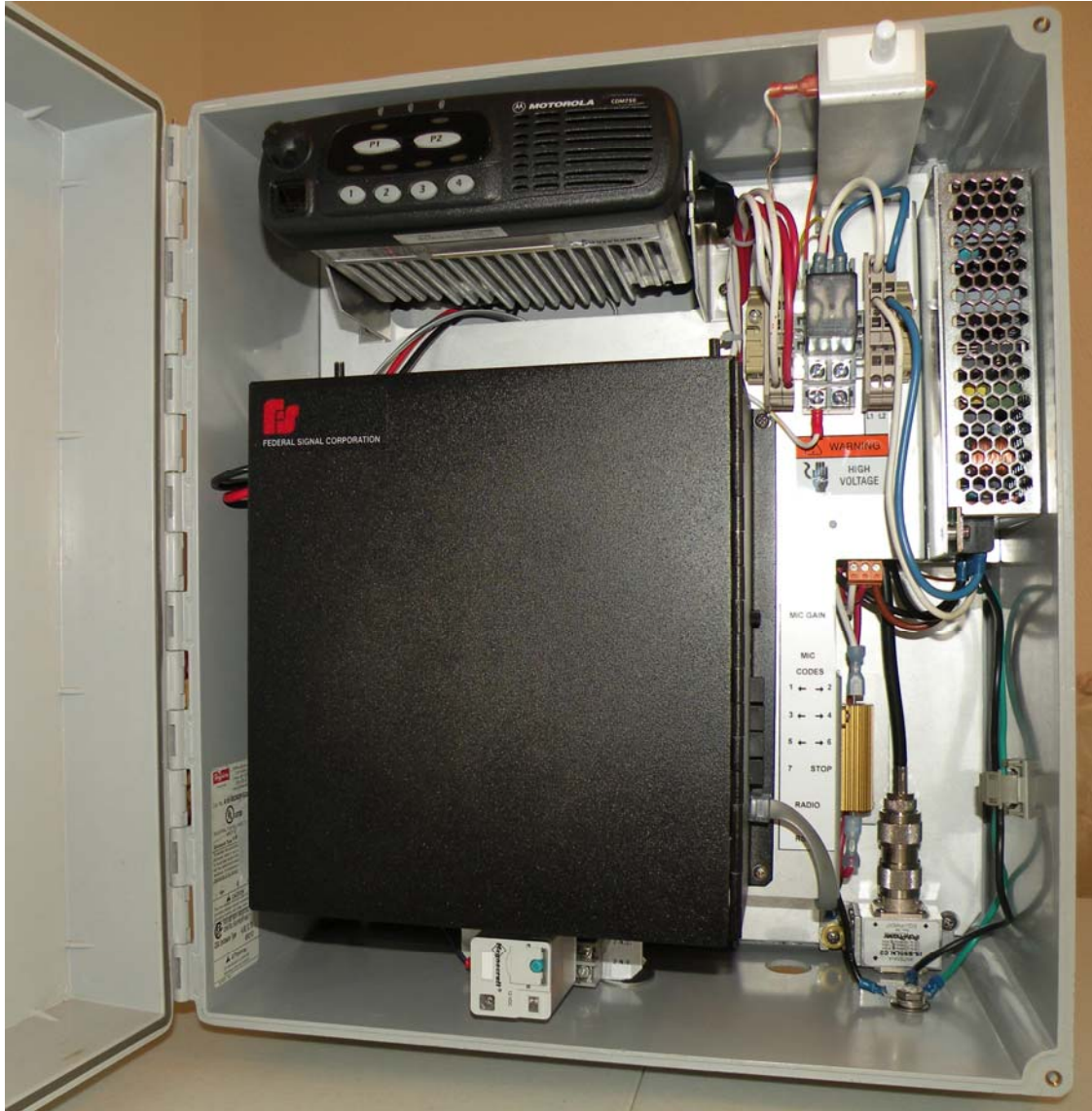
Figure 4.1 – UVRI Inside View
